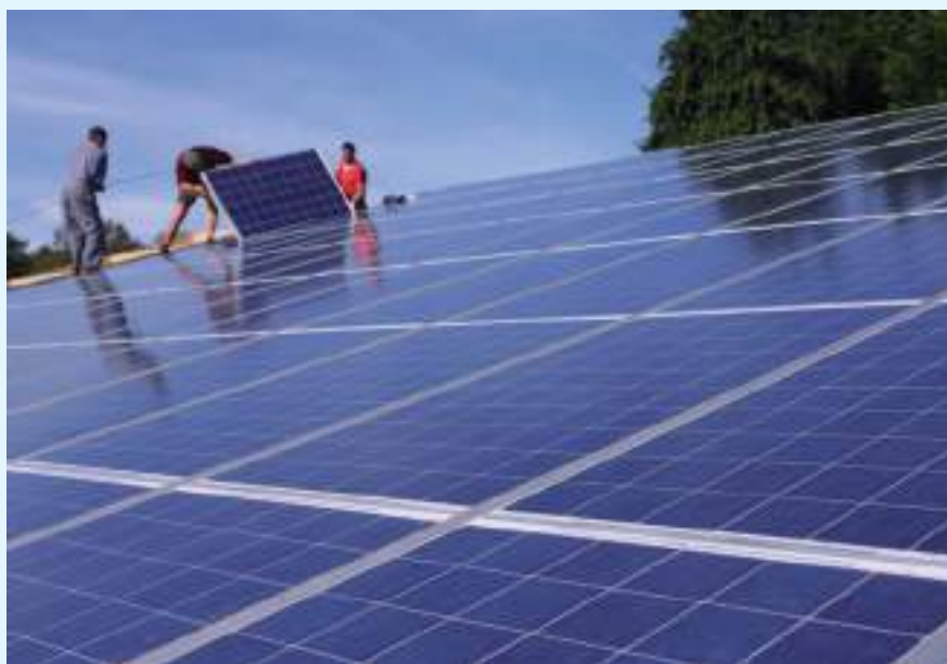
Example of an Integrated PV System (fig. 10)
