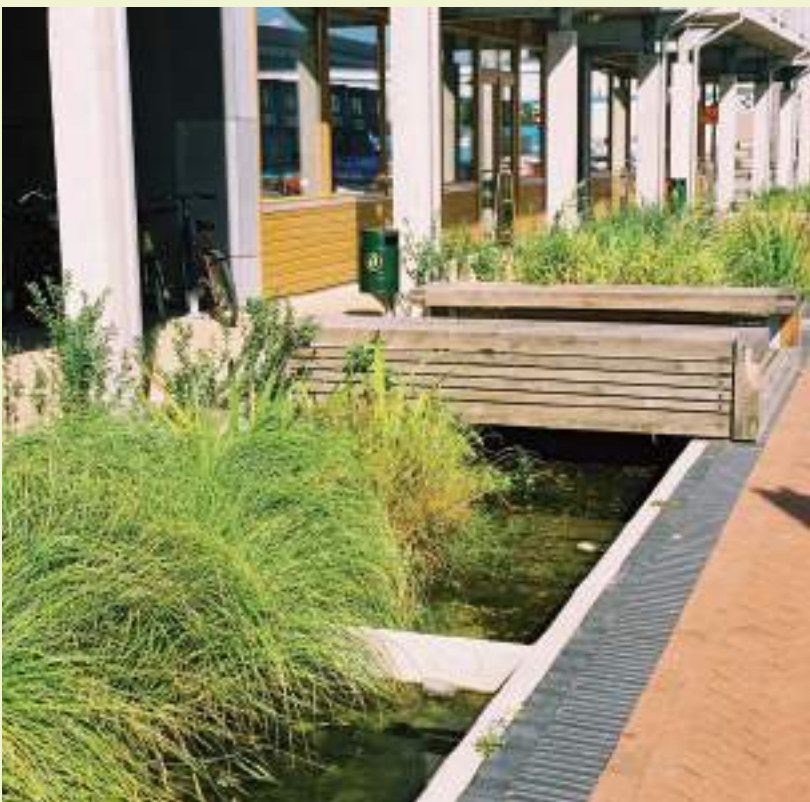
Open rainwater channel (fig. 13)
