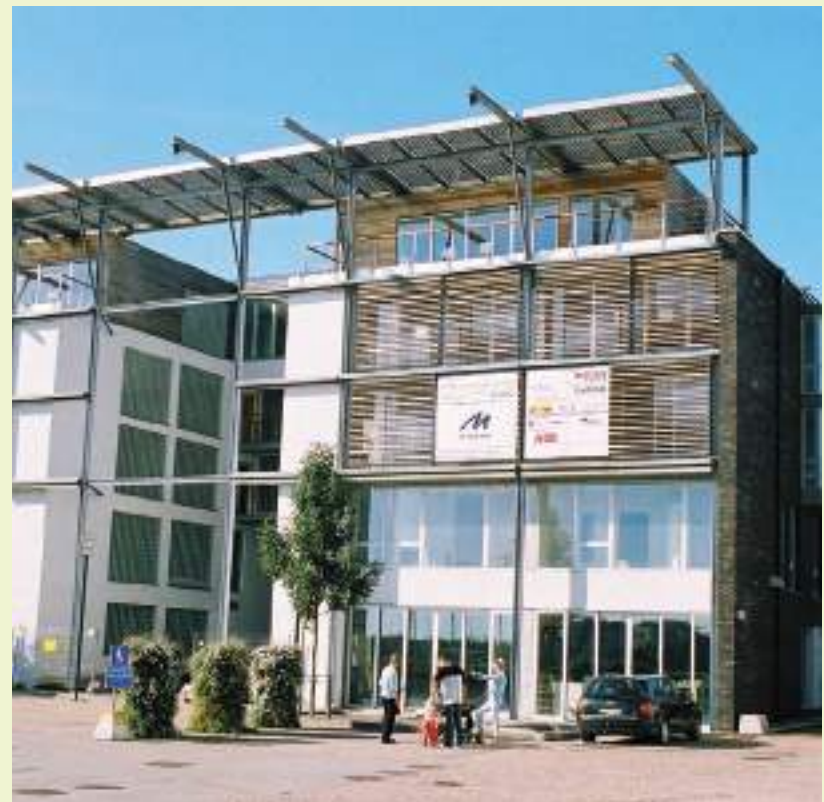
Protecting PV structure (fig. 5)
