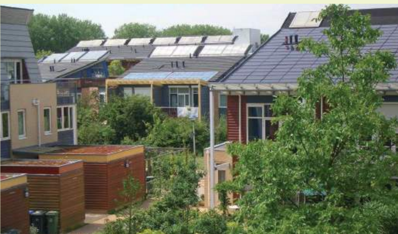
Solar roofs on terraced houses: PVs and solar thermal collectors (fig. 16)
