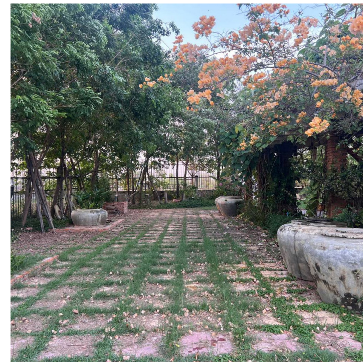
Figure 16. Example of the application of permeable pavement in a parking area in urban Cambodia. Source: Tep Makathy (2025).
