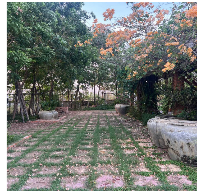
Figure 16. Example of the application of permeable pavement in a parking area in urban Cambodia. Source: Tep Makathy (2025).
